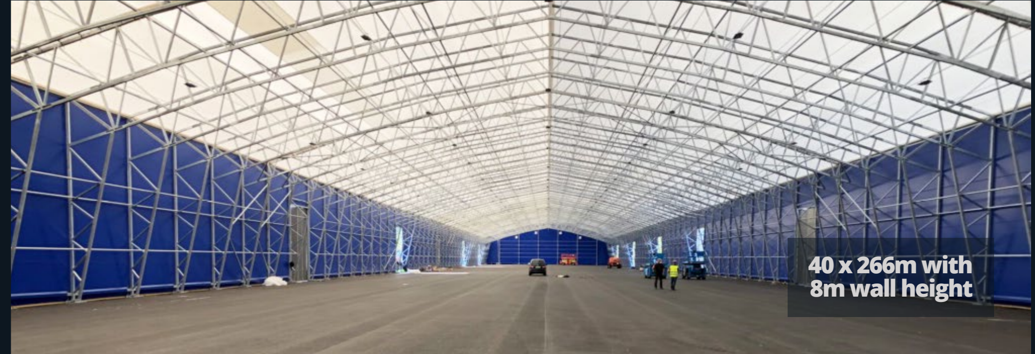
This hall that measures 40 x 266m with 8m wall height required 18.000m 2 of pvc cover and more than 260,000kg of steel
