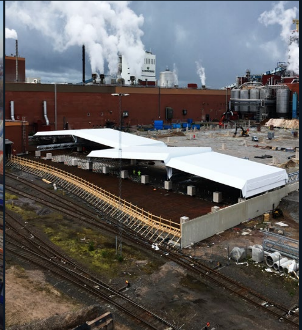
110 meters wide running on a specially designed rails system.
