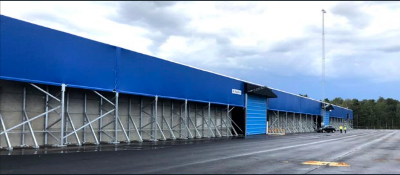
BOTTOM: This hall dimensioned at 40x160m (!) has a concrete rim for storage of wood pellets.
