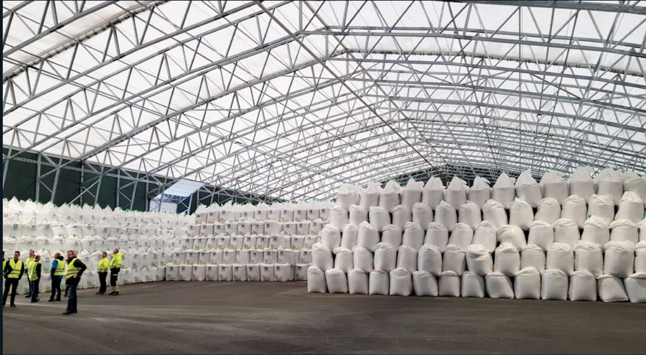
Hall structures for storage and efficient handling of bulk materials.
